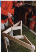
Firm yet flexible. The tabletop is attached with figure-eight fasteners, which allow for seasonal movement.
